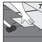
7 If necessary use a tile offset as a tapping block, gently tap with a rubber mallet to ensure edges are well aligned.
