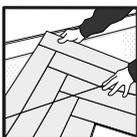
Then using a utility knife or a plunge saw set to 5mm, carefully cut through along the scribe marked line. Retain the offcut triangle for use on the other end of the room.
